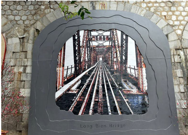
An image of Long Bien Bridge on sealed arch span No. 74
